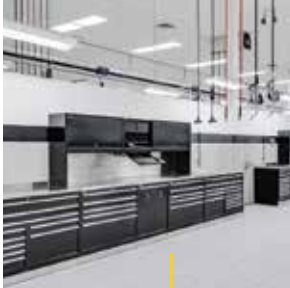
Service Bays & Toolboxes
